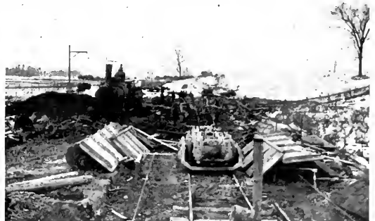
FIG. 11.—CAR BARN AFTER FIRE.
